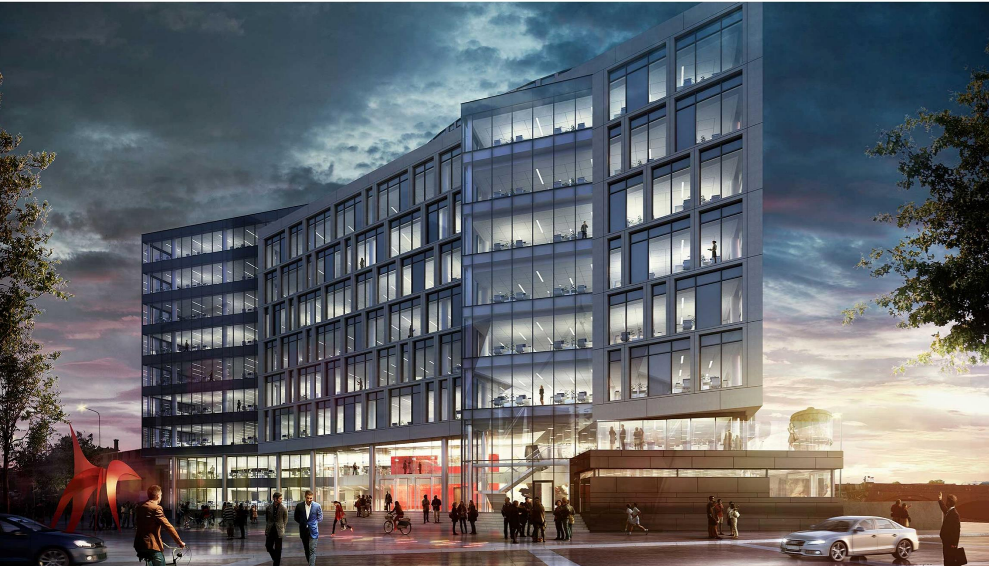
Image by kind permission of Rio Architects
